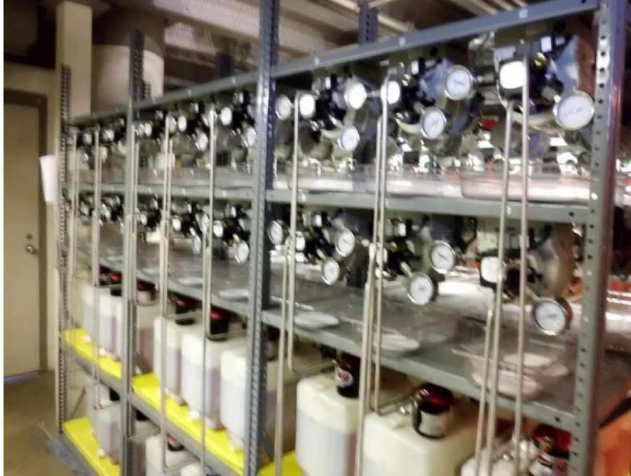
Figure 2-1 Pumps under test at Penn State University
